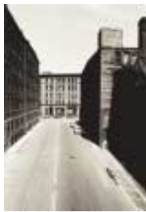
59. Factory street Boston Boston, Massachusetts, 1989. In the city's Back Bay harbor area, I found these old factory buildings, so typical of New England factory architecture of the early twentieth century. I tried to create the mood of a photograph taken around that time, using 35 mm 400 ISO black-and-white negative film. Sadly, when I returned a few years later they had gone.
