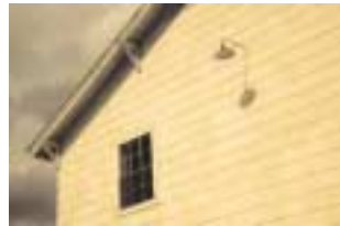
65. corr889_9398 (White barn) Texas, 2003. This white clapboard barn is so typical of rural America. With just the right amount of sunlight casting the shadow of the old-style light fixture, I was able to compose a picture that would express the nostalgic mood I was seeking. I used a Canon 1DS digital camera.
